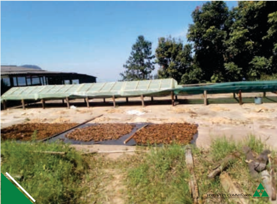
Plate 3.1: Seed drying racks constructed at John Meikle Forest Research Station
