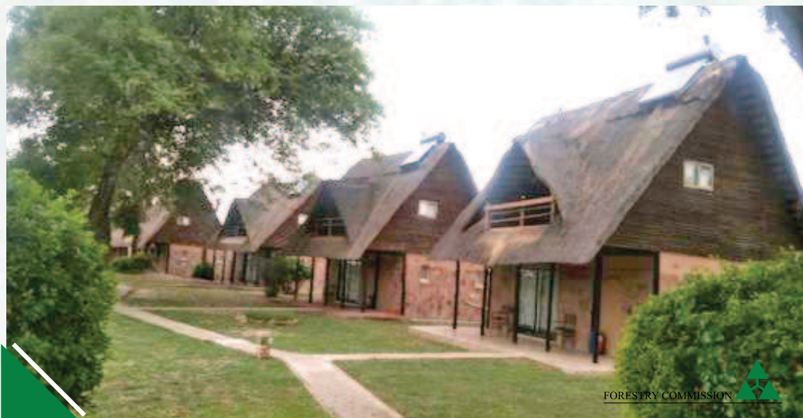
Plate 4.1: Installed Solar geysers at Ganda Lodge.
