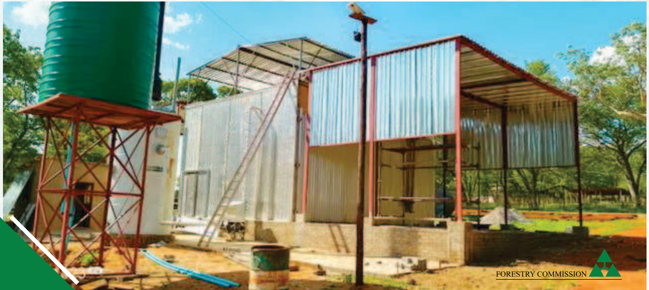
Plate 2.3: Installation of Wood Drying Kiln at Forest Hill, Lupane, Matabeleland North Province.
